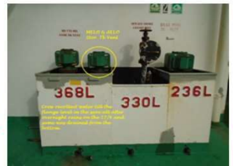
Figure 4 Flange location below the top edge of the save-all coaming
